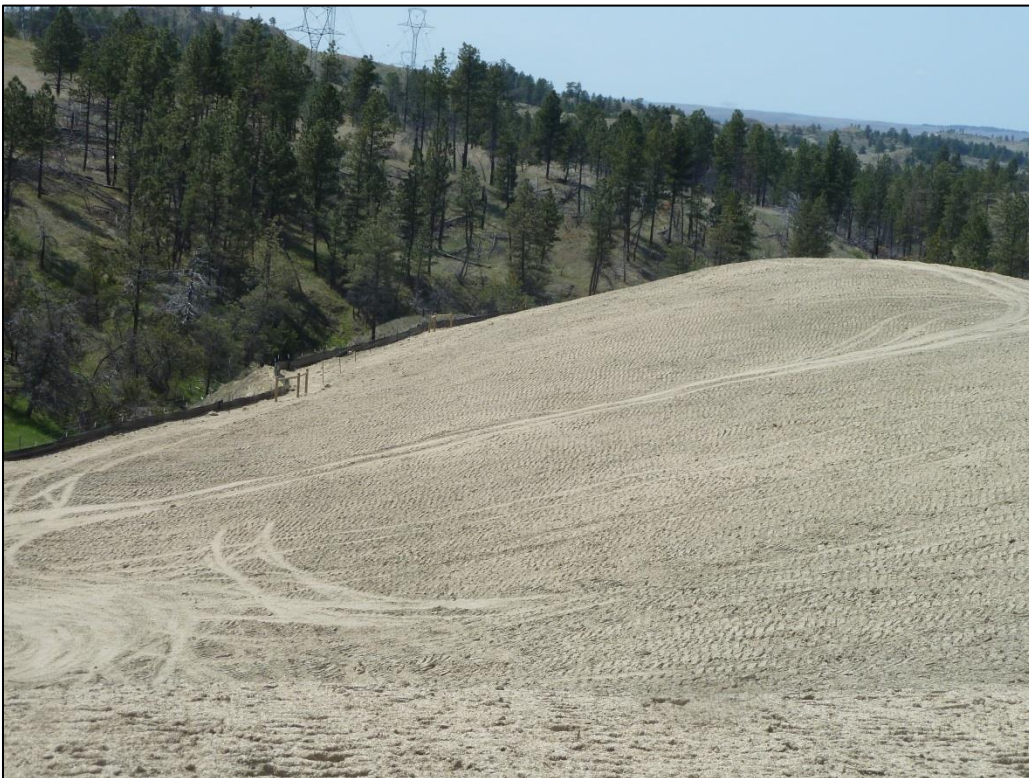
Regrade work (photo taken 5/4/15)
