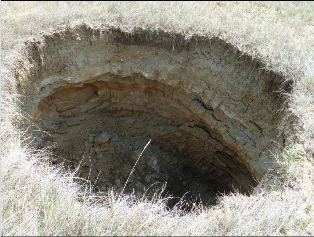
New subsidence feature found at Coal Creek Mine (photo taken 7/1/16)
