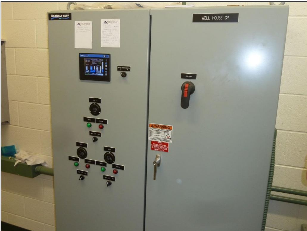
Control panel inside the new Sand Coulee well house (photo taken 6/23/16)
