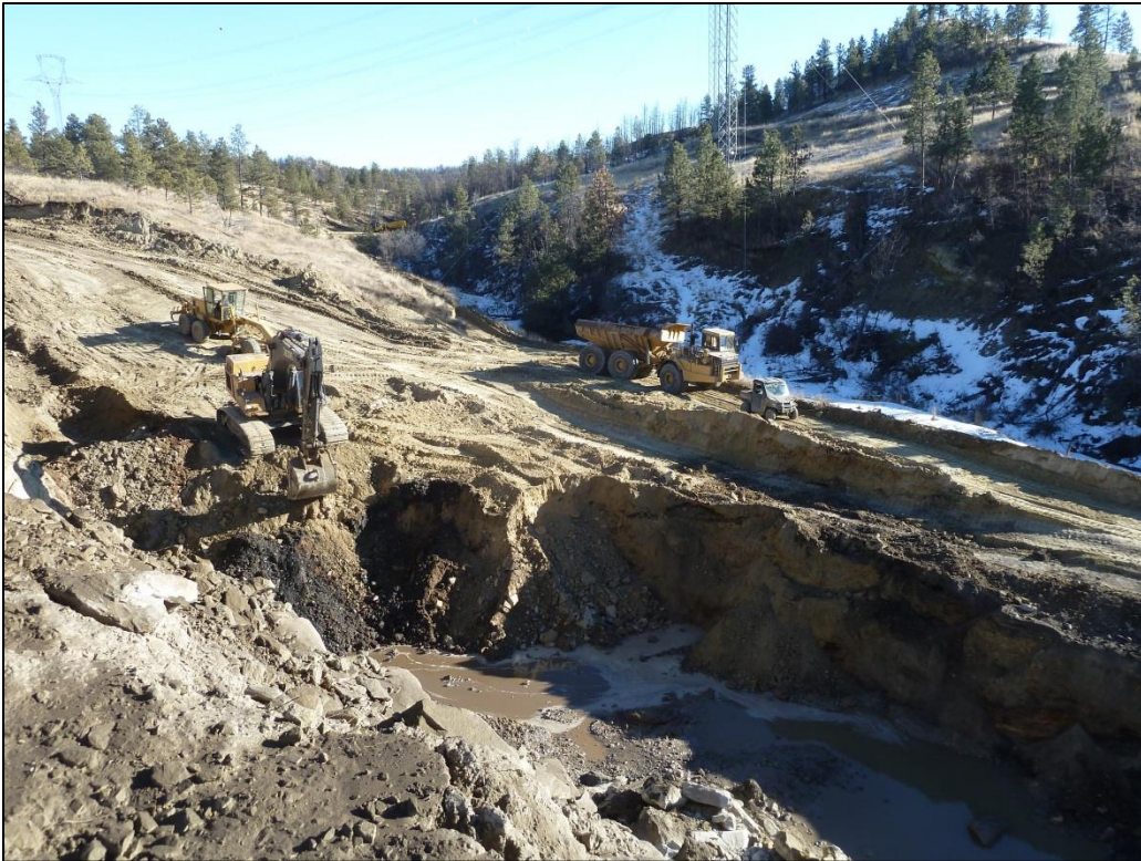
Settlers Stripping Fire Project-work underway on 1/29/15
