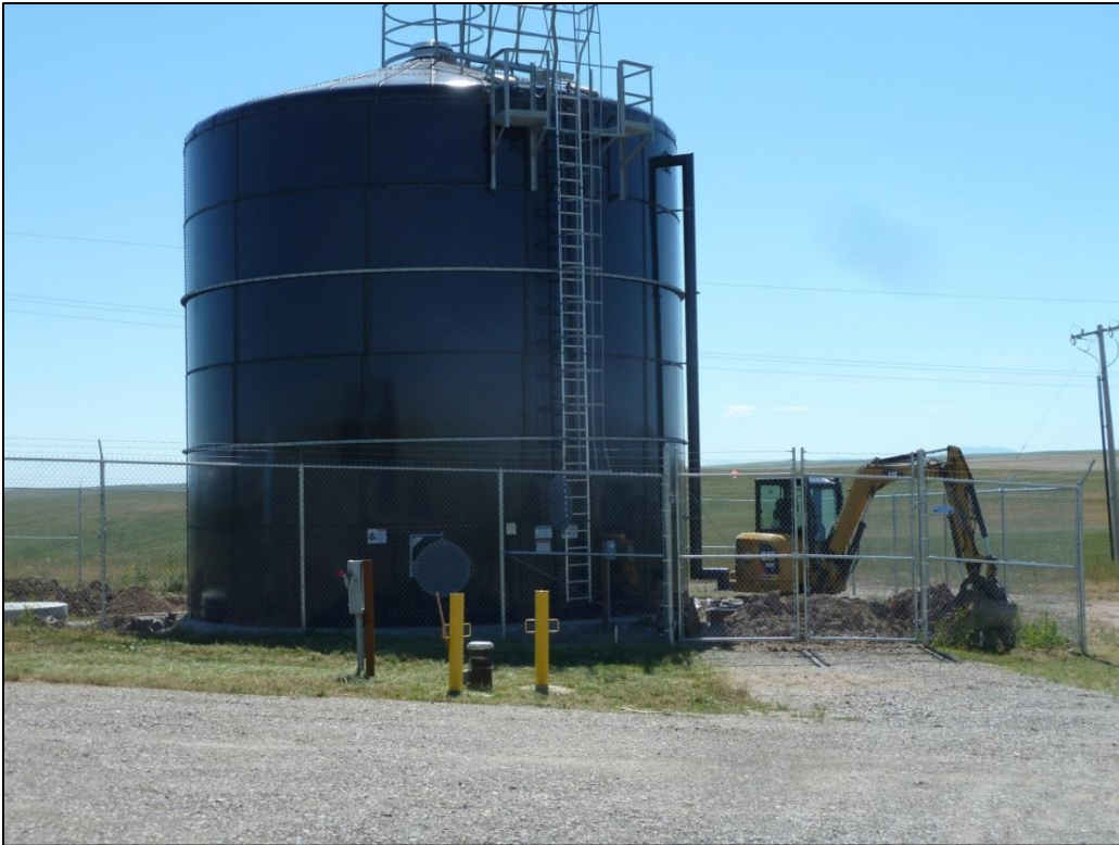
Town of Sand Coulee's new water tank (photo taken 6/23/16)
